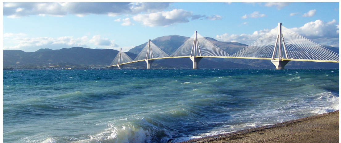
The Charilaos Trikoupis bridge in Greece is an example of a structure engineered to account for seismic activity, the probability of tsunamis as well as the expansion of the Gulf of Corinth due to plate tectonics. During an earthquake, the piers can move laterally on the sea floor with a gravel bed to absorb the energy. The bridge decking is connected to the pylons using jacks and dampers to absorb movement. (Source: Wikipedia)
