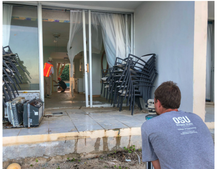
Work for the U.S. Virgin Islands team included an extensive coastal survey of Hurricane Maria's damage to local infrastructure. (Image: Richie Slocum)
