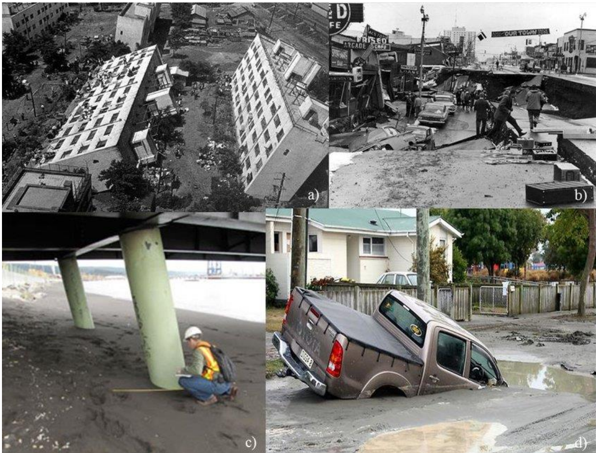
Image 3. Liquefaction-induced damage observed in (a) Niigata, Japan 1964 (From http://civilenggseminar.blogspot.cl ), (b) Alaska, USA 1964 ( http://en.wikipedia.org ), (c) Maule, Chile 2010 (Provided by CGMI Consultants) and (d) Christchurch, New Zealand 2010 (From http://www.news.com.au )
