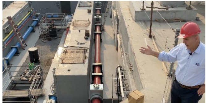
Joel Conte, principal investigator of the NHERI at UC San Diego Experimental Facility shows an overhead view of the Large High-Performance Outdoor Shake Table hydraulic system.
