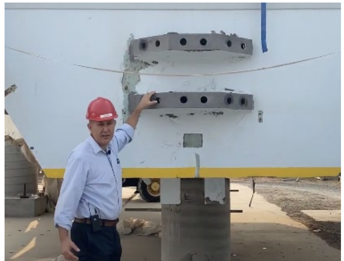
Horizontal actuator connections on the platen.
